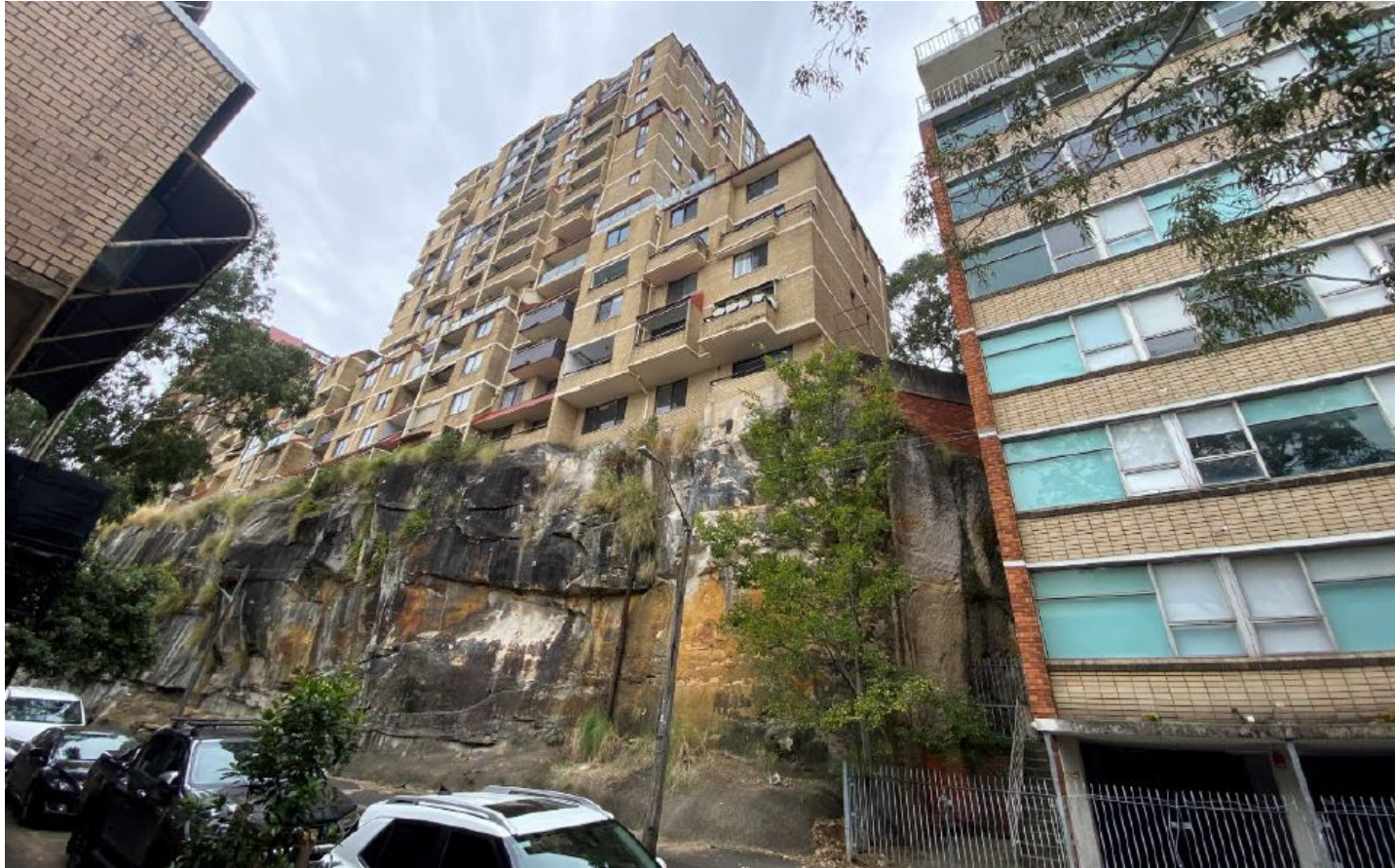
101 – 115 Victoria Street to north
