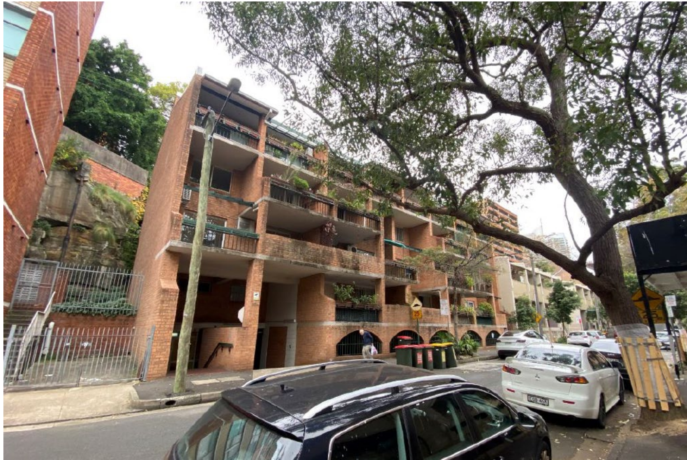
30A – 34 Brougham Street to south
